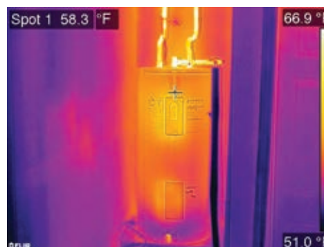
An electric water heater in standby mode has heat loss of 66 degrees.
